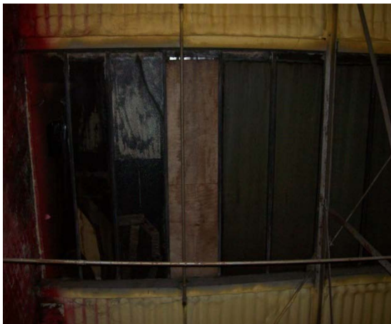
4.01 4 th Floor Goods Lift Lobby Strongly Presumed Woven Rope Seal to Glazing Bars of Northern Roof Light (No Safe Access)
