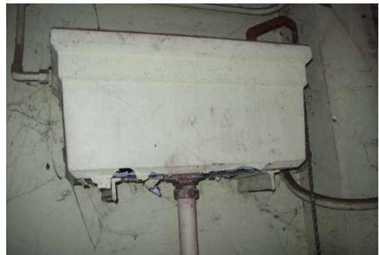
Sample No: 18/2/B/14/JPS8 1.07 First Floor Redundant Toilet Thermoplastic Cistern
