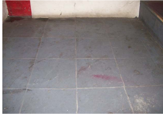
As Sample No: 18/2/B/14/JPS4 1.01 First Floor Circulation Area/Stairwell Vinyl Floor Tiles and Bitumen Adhesive
