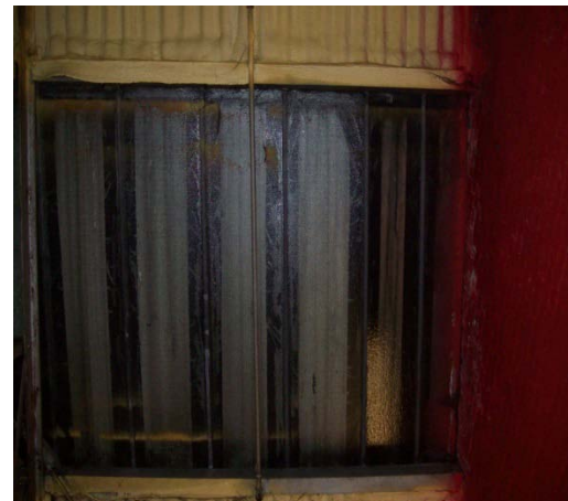
4.01 4 th Floor Goods Lift Lobby Strongly Presumed Woven Rope Seal to Glazing Bars of Northern Roof Light (No Safe Access)
