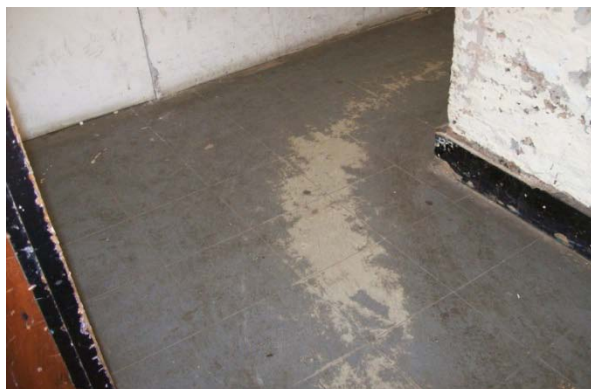
Sample No: 18/2/B/14/JPS4 G.05 Ground Floor Circulation Area/Stairwell Vinyl Floor Tiles and Bitumen Adhesive
