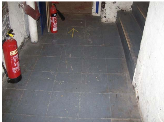
As Sample No: 18/2/B/14/JPS4 2.01 2nd Floor Circulation Area/Stairwell Vinyl Floor Tiles and Bitumen Adhesive
