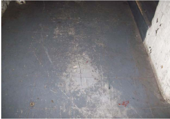
As Sample No: 18/2/B/14/JPS4 1.01 First Floor Circulation Area/Stairwell Vinyl Floor Tiles and Bitumen Adhesive
