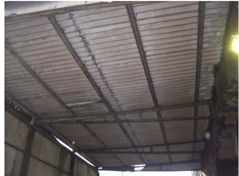
As Sample No: 18/2/B/14/JPS1 Ex.1 Ground Floor External Canopy Loading Area Corrugated Cement Roof
