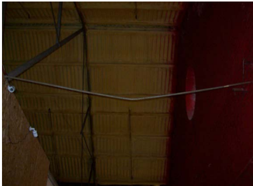
Sample No: 18/2/B/14/JPS13 4.01 4 th Floor Goods Lift Lobby Spray Foam Insulation Covered Corrugated Cement Roof Sheets
