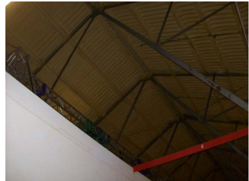
Sample No: 18/2/B/14/JPS13 4.01 4 th Floor Goods Lift Lobby Spray Foam Insulation Covered Corrugated Cement Roof Sheets
