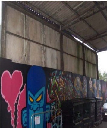
Sample No: 18/2/B/14/JPS1 G.01 Ground Floor Goods Lift Lobby Corrugated Cement Roof
