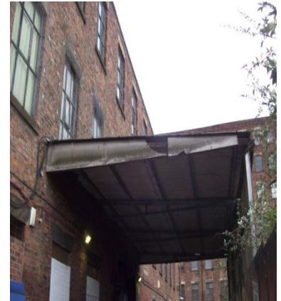
As Sample No: 18/2/B/14/JPS1 Ex.1 Ground Floor External Canopy Loading Area Corrugated Cement Roof
