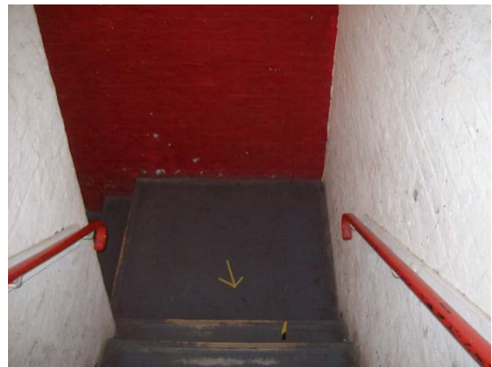
As Sample No: 18/2/B/14/JPS4 2.01 2nd Floor Circulation Area/Stairwell Vinyl Floor Tiles and Bitumen Adhesive
