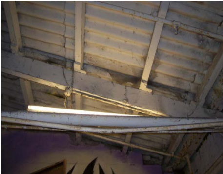
Sample No: 18/2/B/14/JPS1 G.01 Ground Floor Goods Lift Lobby Corrugated Cement Roof
